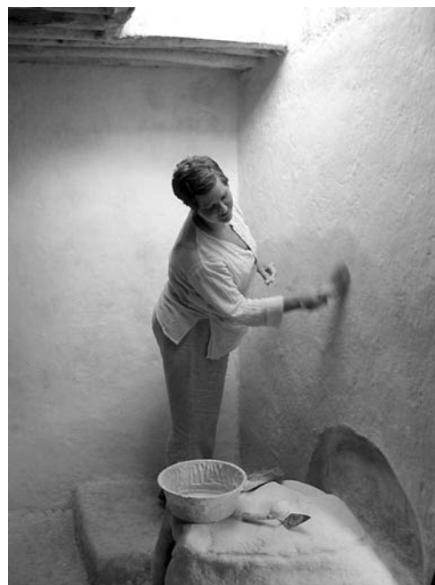
Figure 23.6. Burnishing plaster layers with a grass brush.
