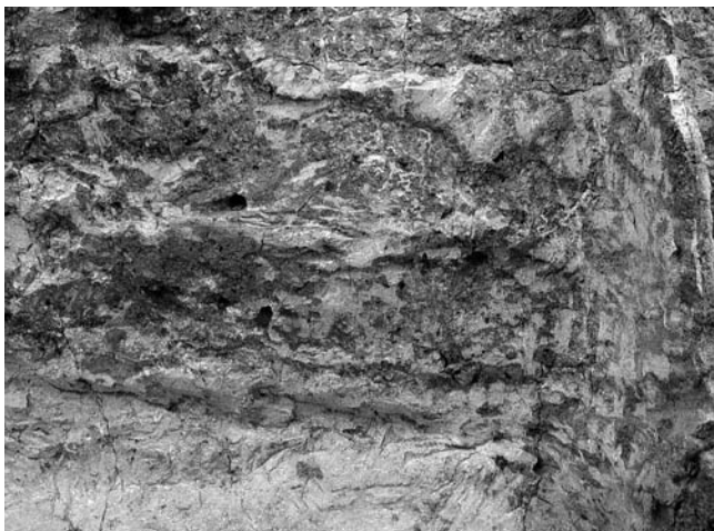
Figure 5.11. The rippled wall plaster applied to the southern partition wall (F.161).
