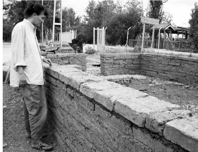
Figure 2.13. Mirjana Stevanović inspects the mud-brick walls of the Replica Neolithic House in the early stages of its construction in 1999.
