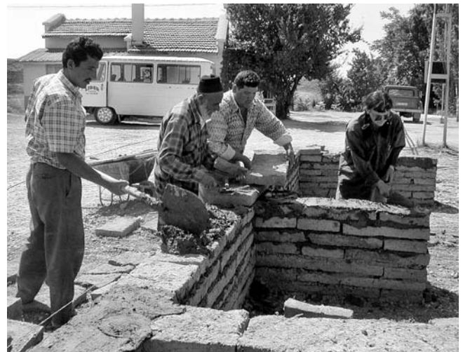
Figure 22.11. Laying the walls.
