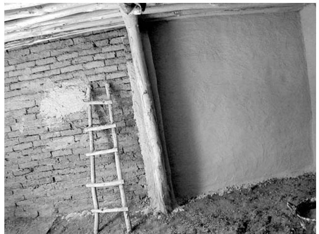
Figure 22.31. Application of the preparatory layer of plaster.
