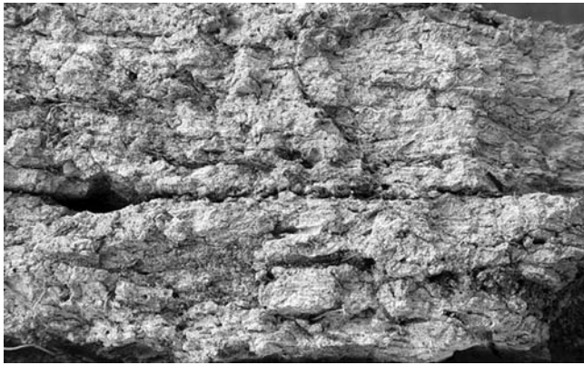
Figure 5.10. Multiple layers of wall plaster in Building 3.
