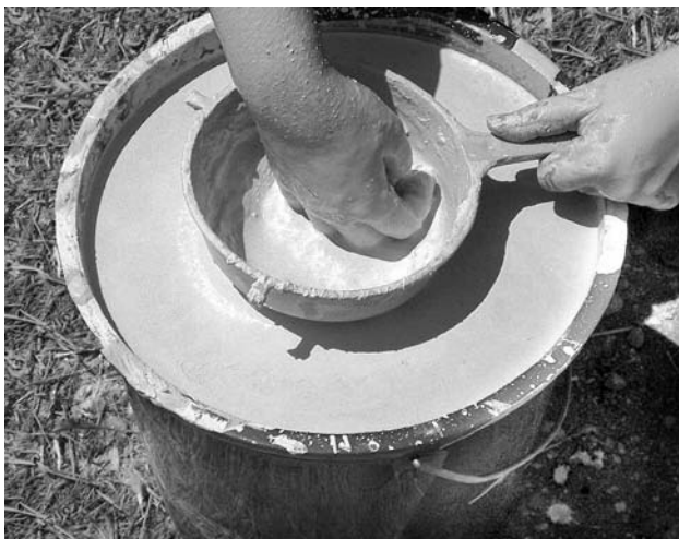
Figure 23.5. Detail of sifting plaster through a sieve.
