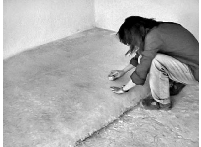
Figure 22.34. Burnishing the plaster on the house platform.
