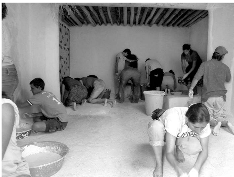
Figure 22.32. Application of the finishing coats in the house interior.
