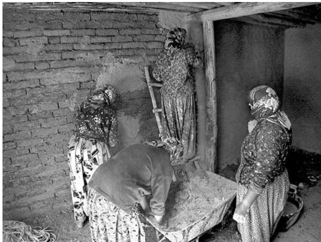
Figure 22.30. Interior plastering.
