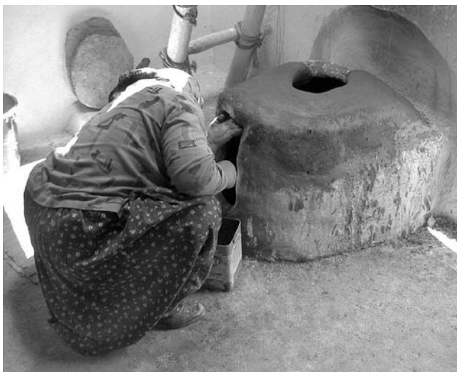
Figure 22.22. Oven opening under construction.
